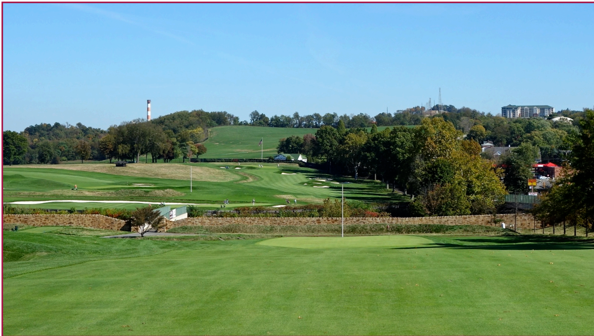
Hole 1 and the Turnpike wall are located in the foreground, while Hole 2 and the east part of the golf course is now visible in the distance.
